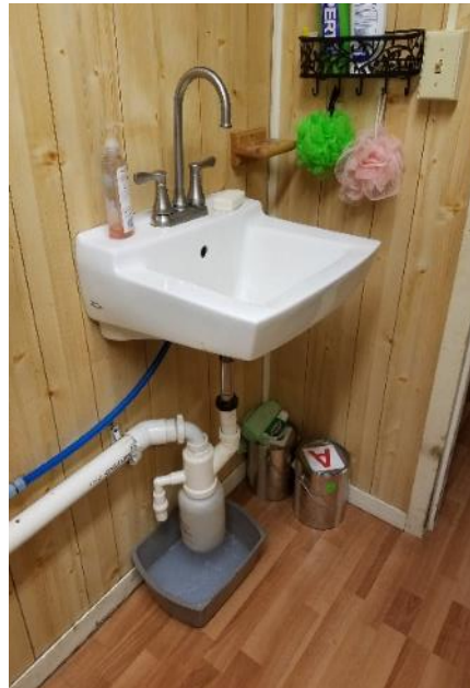
Low-flow gravity-fed sink and drainage
