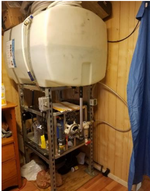
Water treatment unit and storage tank
